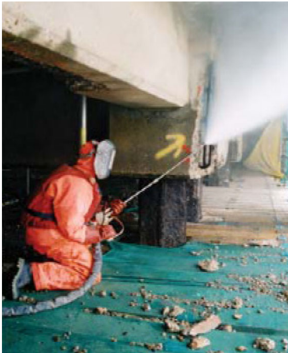
Left: Hydrodemolition (stock photo)
