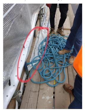
On investigation it was found that the scaffold fan had not been constructed in accordance with the scaffold design drawings and it was not double boarded.
