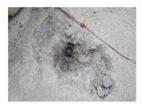
The operative accidentally damaged the anode with the breaker. The damage exposed the battery to the atmosphere and caused it to catch fire.
