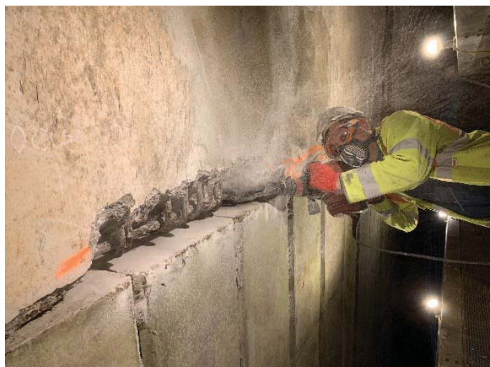
Half-Joint Repairs
