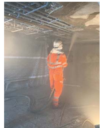
Concrete Spraying
