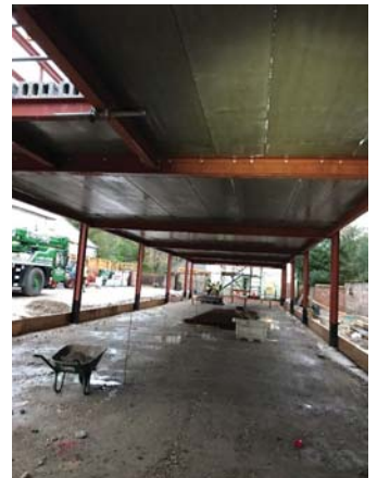
Steel Frame Erected Along with Hollow Core Flooring at First Floor Level
