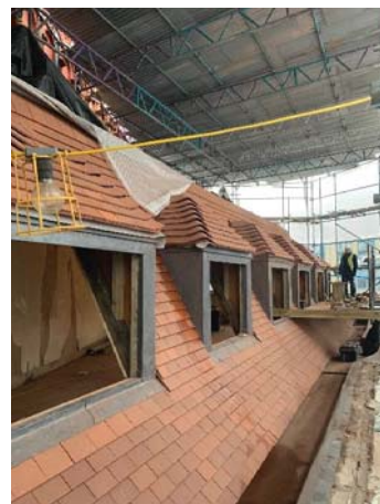
Tiling of Existing Roof at Roof Level
