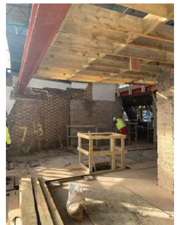
9m Span Beam to Support Green Roof at Roof Level
