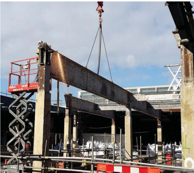
Demolition of the original roof
