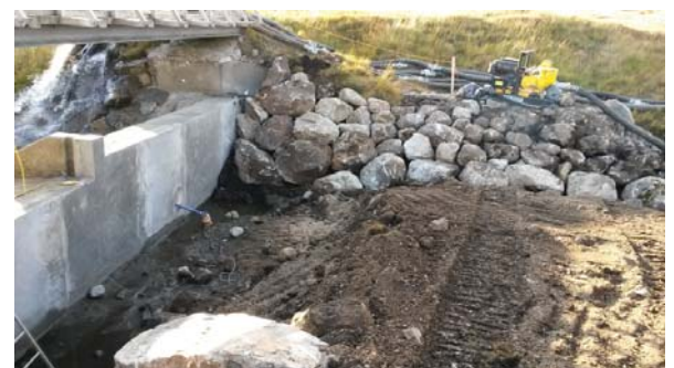
Replacing the stone rip-rap
