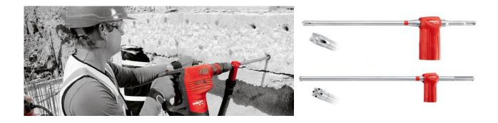
"These Hilti TE-CD hollow drill bits have been used on various CRL sites and 'do what they say they will do' - reduce the production of air-borne dust, utilising the purpose designed sleeve on the shank, attached to a class M vacuum.
