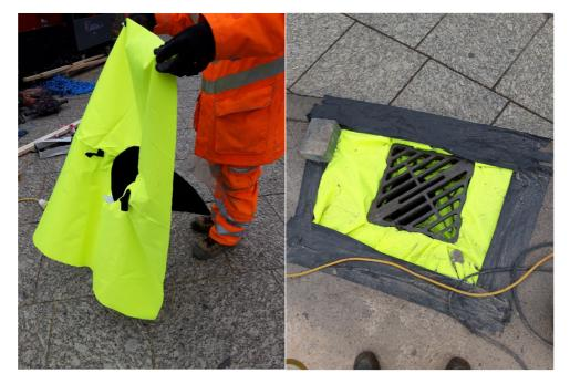
Two types are available, either sediment (retains up to 21kg sediment) or oil and sediment filters (retains up to 19kg of sediment and 1 litre of hydrocarbon).
